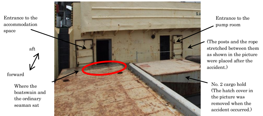
Photo 3: Entrance to Accommodation Space and Entrance to Pump Room
