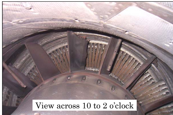
Photo 4 Damage viewed from Engine Exhaust
