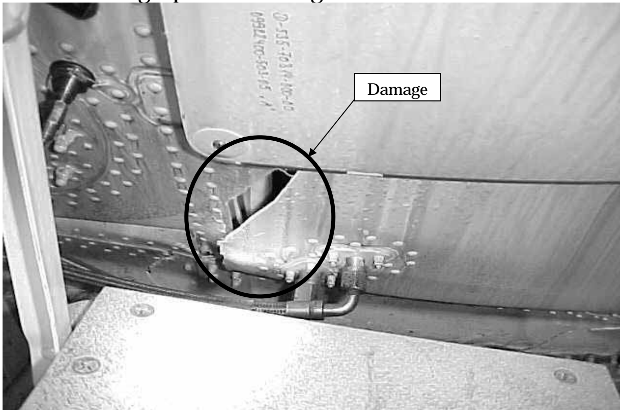
Photograph-5: Damage of the Aft Bulkhead
