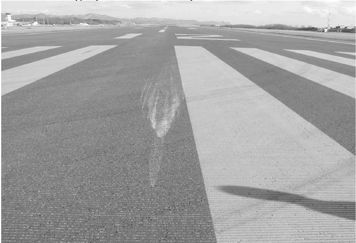
Photograph-2: The scrape marks on RWY 12
