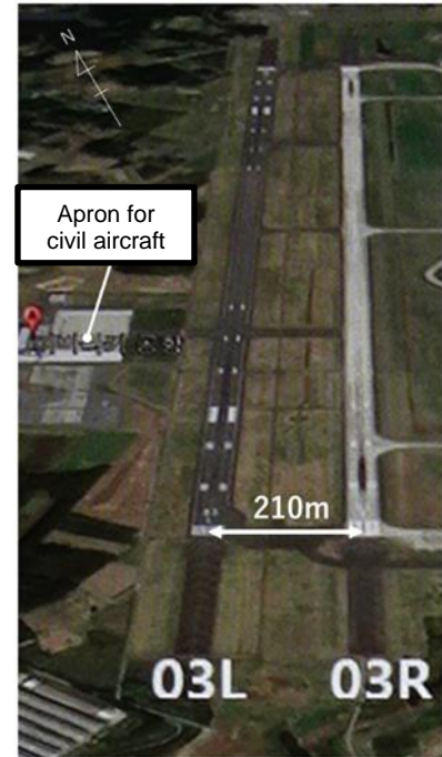
Figure 2: Hyakuri Airfield Runways (Source: Eastar Jet Co., Ltd.)
