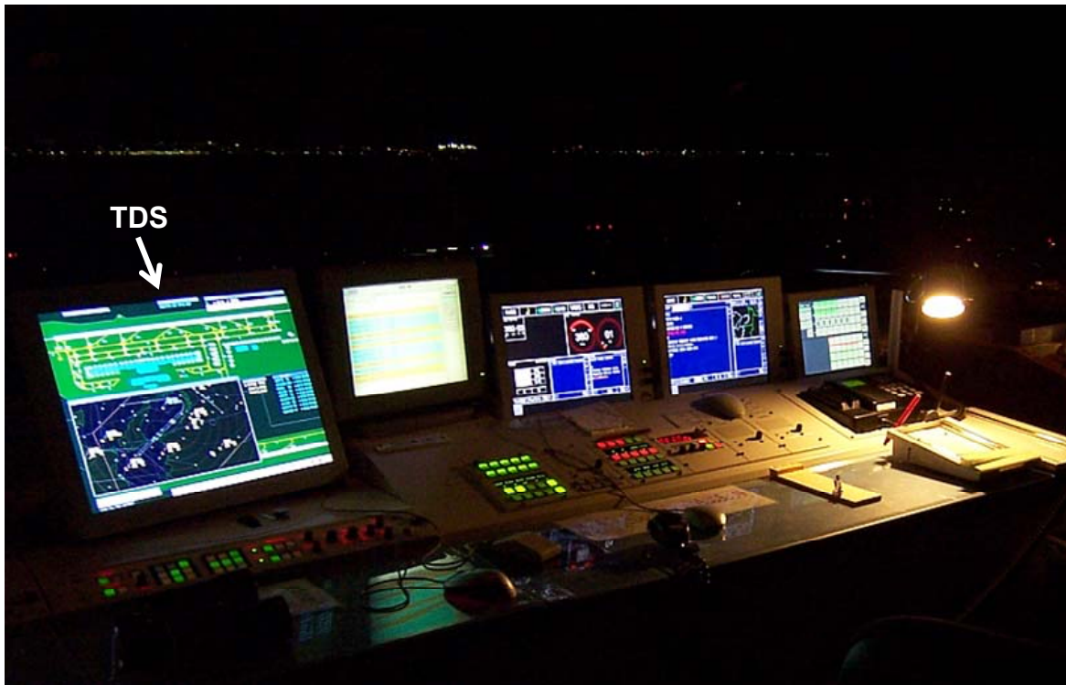
Photograph 1 Control Tower (Runway-A side)
