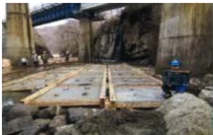
Figure 21: Installation of new riverbed protection blocks (completion of concrete placement)
