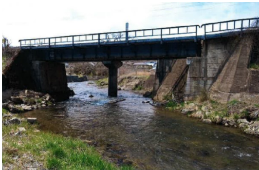
Figure 17: No.4 Kitakami River Bridge (Full view from the upstream side)
