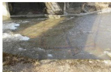
Figure 23: Completion of work (riverbed bottom)
