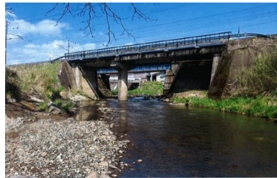
Figure 18: No.4 Kitakami River Bridge (Full view from the downstream side)
