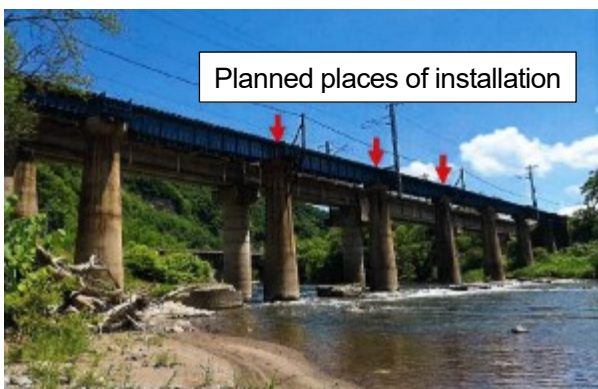
Figure 19: No.8 Mabechi River Bridge (Full view from the downstream side)
