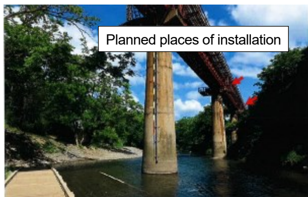
Figure 20: No.10 Mabechi River Bridge (Full view from the downstream side)
