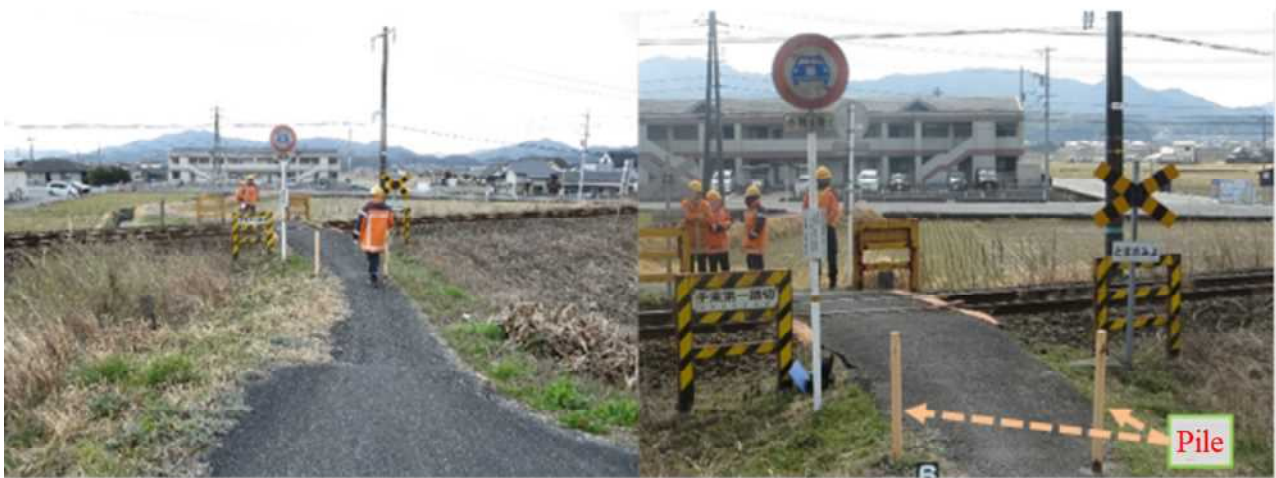
Photo 1. Status of level crossing viewed from the entered bicycle
