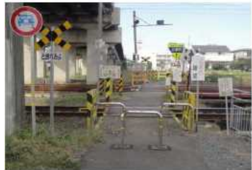
Example of installation of the fence to stop passersby riding bicycles
