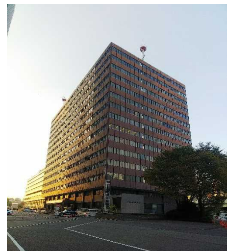
Central Government Otemachi Building No. 3
