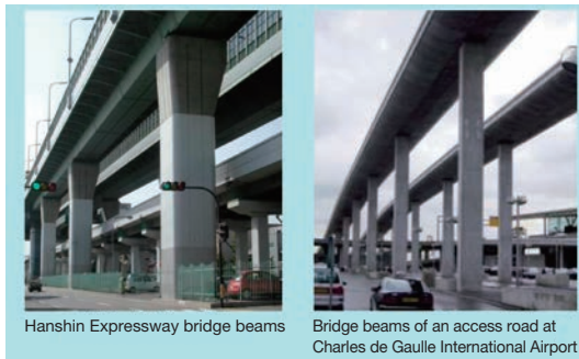
Comparisons of Bridge Beams in Japan and France
