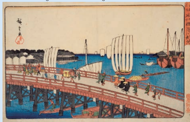
Figure 1-1-10 Eitai Bridge in the Edo Period
