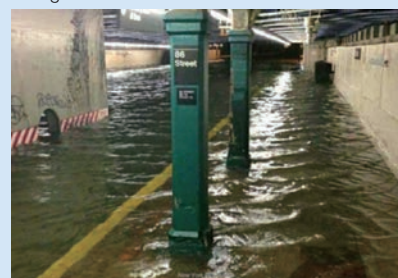
Figure 1-2-26 86th Street Station Flooded
