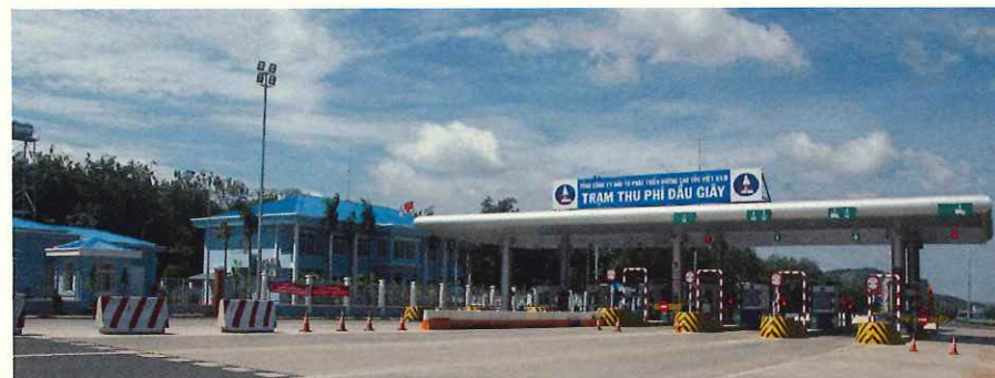
南北高速道路ホーチン〜ゾーサイ間 ITS工事完工 / North-South Expressway ITS construction
