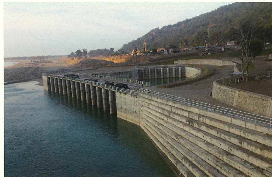
灌漑頭首工工事(ネパール) / Construction of irrigation weir (Nepal)
