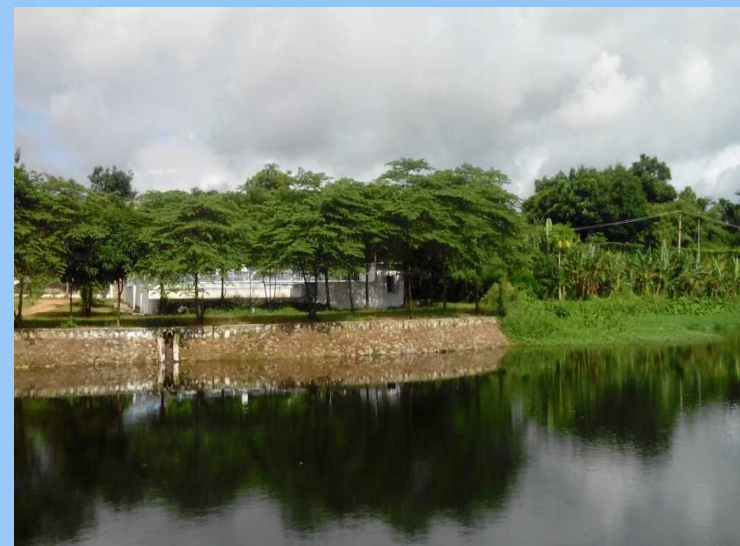
TREATED WATER COLLECTION OR RETENTION POND
