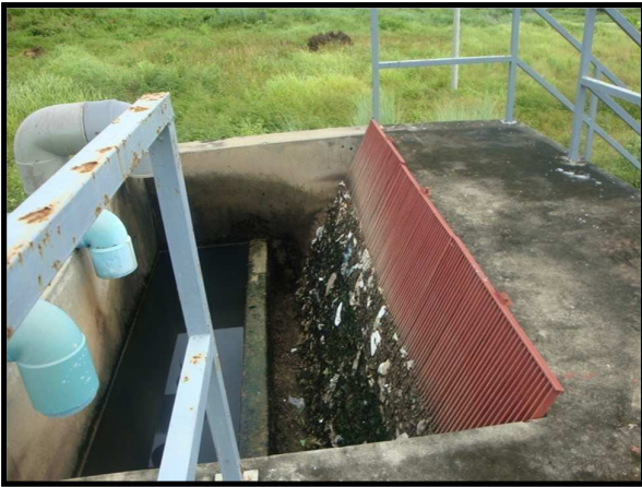
GRIT CHAMBER (INLET OF SEWAGE TREATMENT PLANT)
