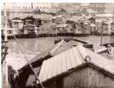
Illegal construction along a river
