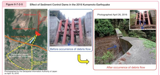
Houses, hospitals, a national road, and other structures in the sediment disaster hazard area were protected from a sediment disaster by the sediment control dam.
