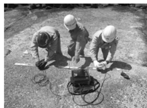
護岸の点検・補修
