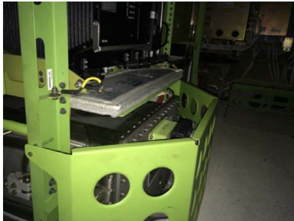
Conditions surrounding the battery enclosure
