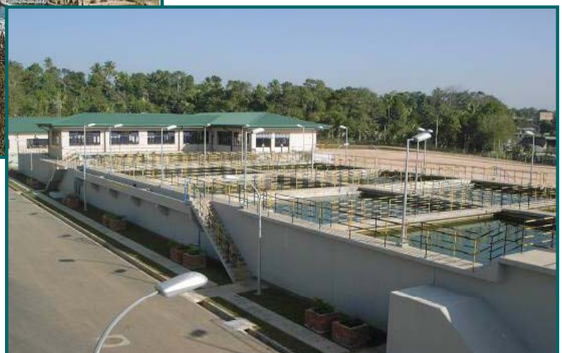
Kandy water plant Capacity: 36,600m 3 /day (2006, Sri Lanka)
