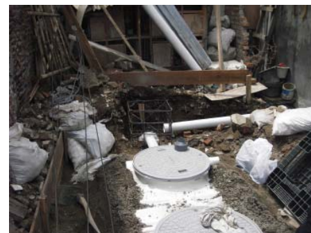
Backfilling
