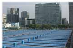
Shibaura water reclamation center, Tokyo
