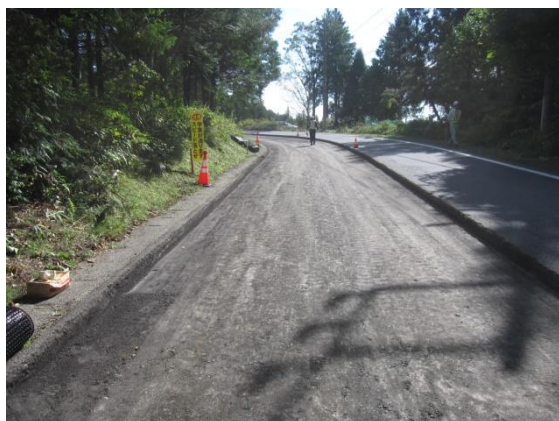
(a) 舗装の切削
