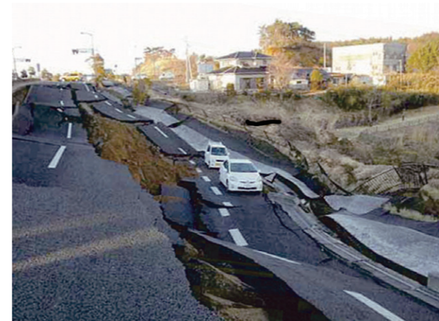
On March 11, 2011 a massive earthquake and the following giant tsunami caused an enormous amount of damage to the roads in Japan (National Highway 6, Hirono-machi, Fukushima Prefecture) (Photo: Tohoku Regional Development Bureau)
