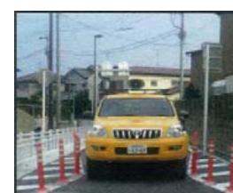
Road narrowing fence
