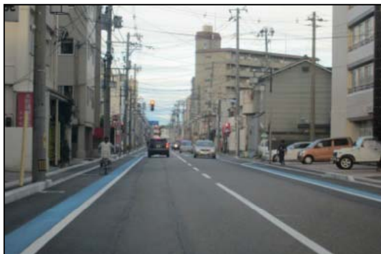
Colored road shoulder
