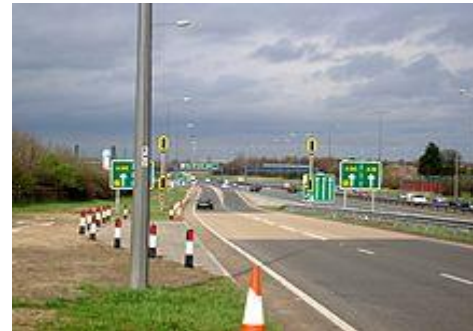
Ramp Metering on the A19 in Middlesbrough (United Kingdom)
