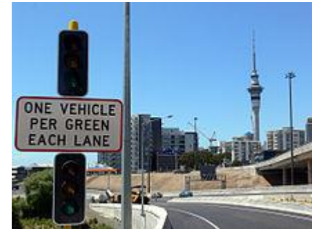
Ramp metering on North Western to Northern connection in Auckland. (New Zealand)
