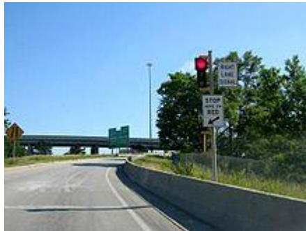
A Milwaukee, Wisconsin ramp metering (USA)
