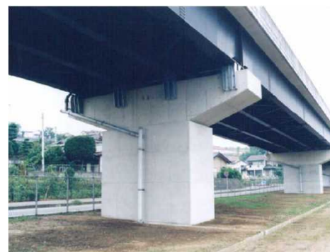
橋梁の耐震補強
