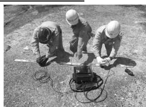
護岸の点検・補修
