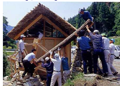
Restoration of a water wheel
