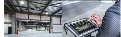
LED lights are used in the overall facility, permitting reduction of running cost.
