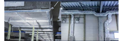
Air inlet in the underground base-isolation pit.
