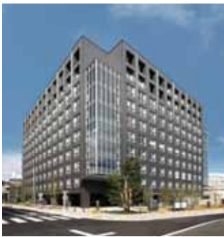
大津地方合同庁舎 Otsu National Government Building
