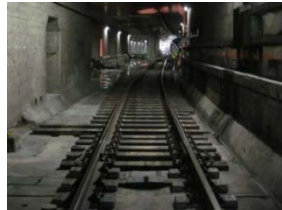
◀A線既設分岐器撤去(H23.5)▶
